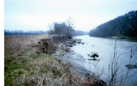
Figure 6. Erosion on left bank of Neosho River just downstream from riprap at Oswego overflow dam. Location of Oswego overflow dam shown in figure 2.
